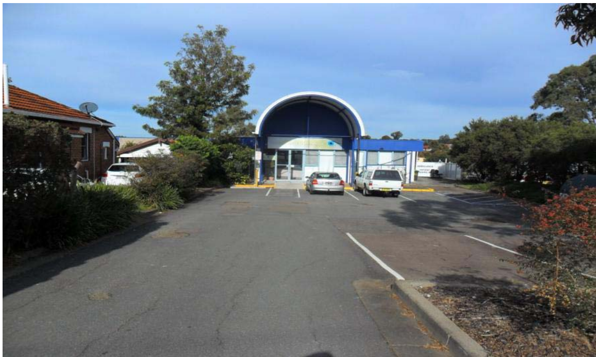
Photo 2: Northern perspective of existing hospital facility from Christo Road
