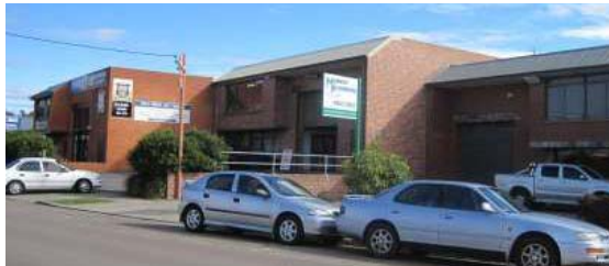
Photograph 4: View looking west along Mitchell Street
